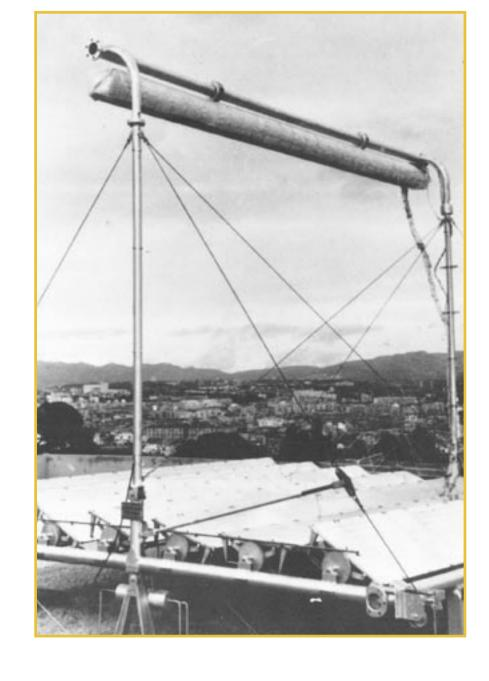
Fig. 6 –The first Fresnel Linear Reflector, pioneered by Giovanni Francia and installed in cooperation with Marcel Perrot in Marseilles in 1963 - 1964 (Photo courtesy of the Francia heirs).
