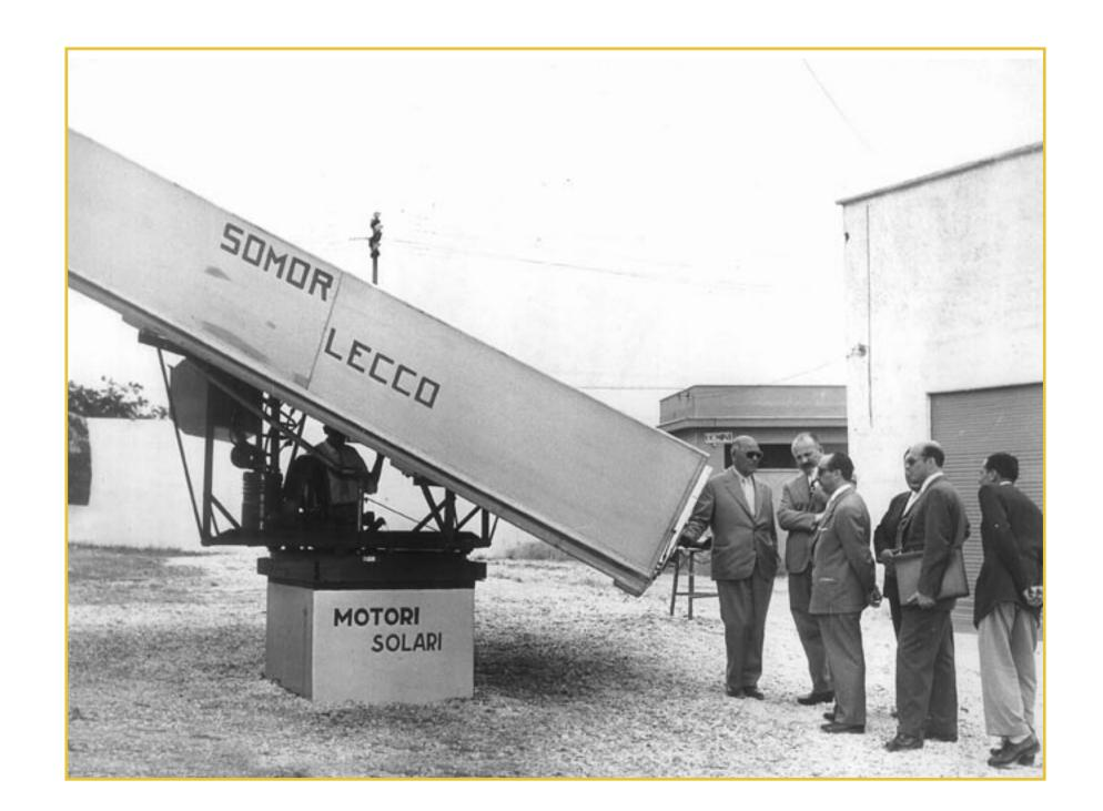
Fig. 2 – The Somor Solar Pump invented in 1948 and patented in 1951 by Ferruccio Grassi from Lecco (Italy). Somor Pump was exhibited in Phoenix (Arizona, USA) in 1955 on the occasion of the 1st Solar World Symposium organized by the Association of Applied Solar Energy (AFASE), the precursor of the International Solar Energy Society (ISES) (Photo courtesy of the Grassi heirs).
